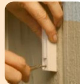
Then remove your doorbell from the wall, and disconnect the wires.
