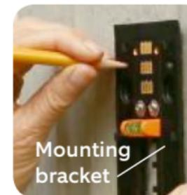
Then **remove the orange tape**, and use the mounting bracket as a template to mark the four corner holes.
